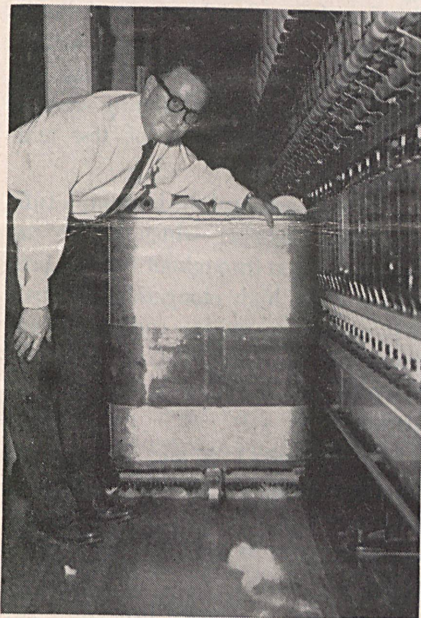
John M. Morrow demonstrates use of his newly-patented floor-sweeping brush mounted beneath a roving box.
