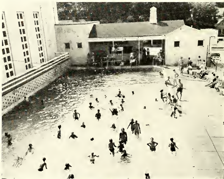
Community Center Swimming Pool
