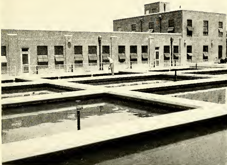
Concord's Modern Water Filtering Plant
