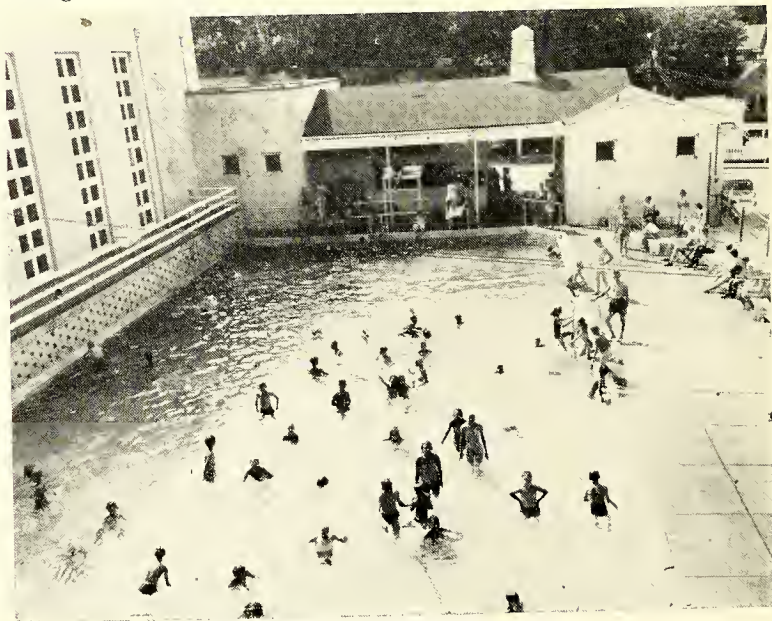
Community Center Swimming Pool
