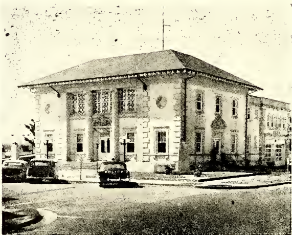
The Morehead City Municipal Building
