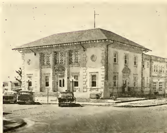
The Morehead City Municipal Building
