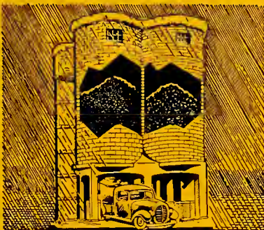
"COAL FROM SILOS"
