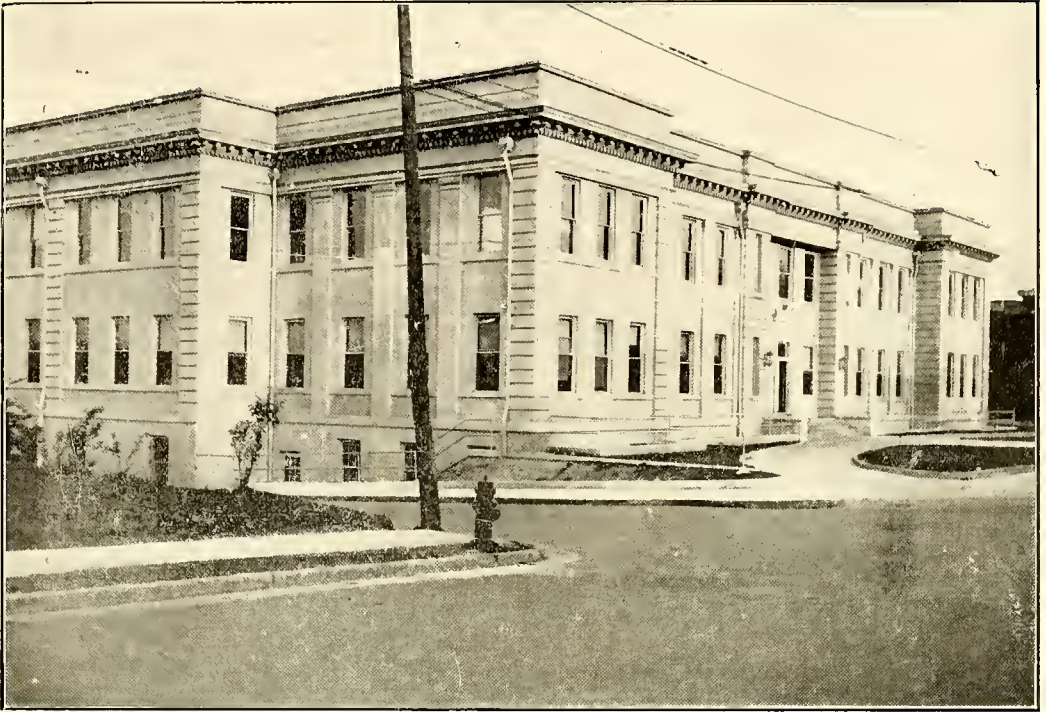
View of City Hall
