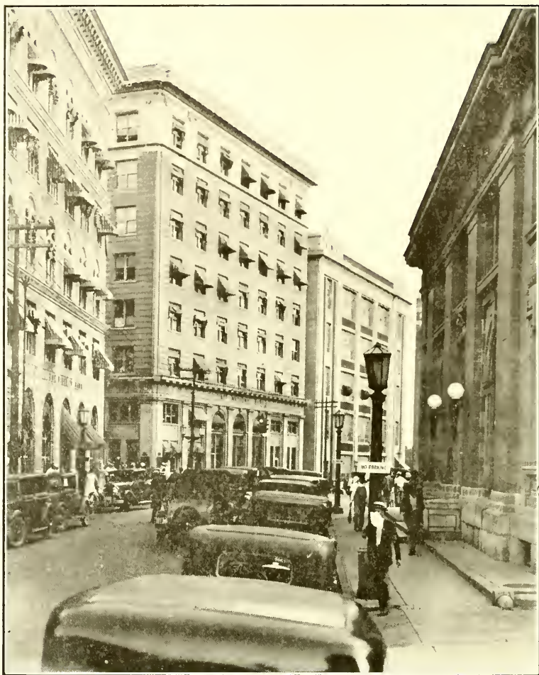
VIEW OF CORCORAN STREET, LOOKING SOUTH
