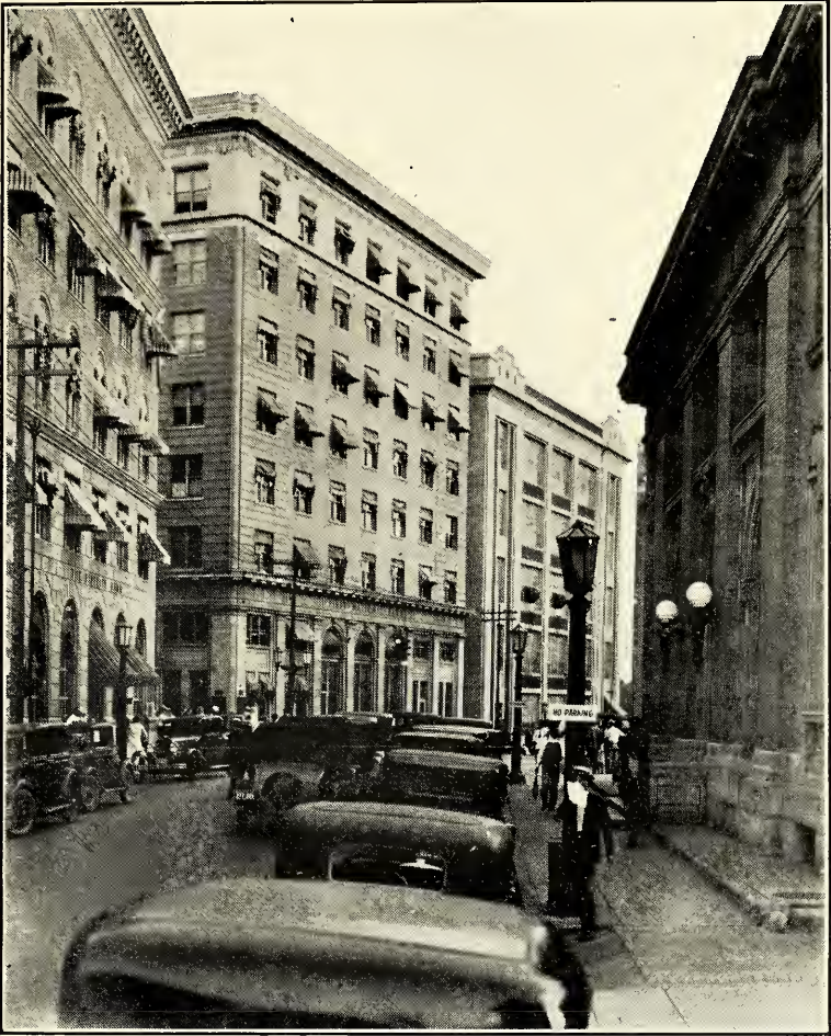
VIEW OF CORCORAN STREET, LOOKING SOUTH
