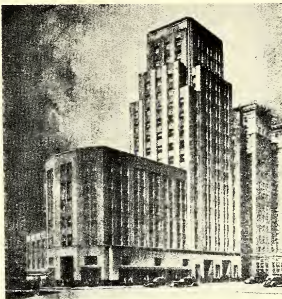
View at One Eleven Corcoran Street, Constructed at a Cost of $1,000,000, in the Heart of Durham's Business District
