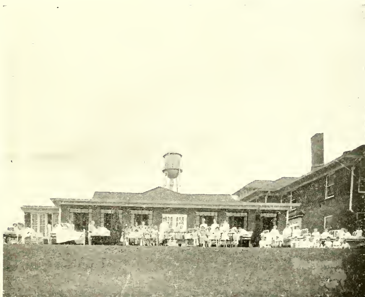
Partial View of North Carolina Orthopedic Hospital
