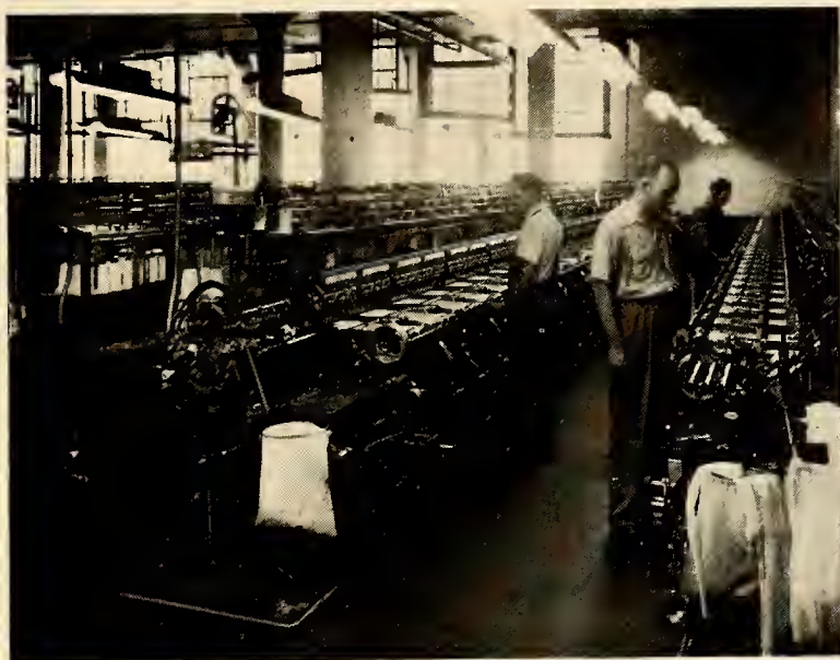
Men and Machines at Work in One of 33 Hosiery Mills, with Daily Capacity of 50,000 Dozen Pairs of Hose.
