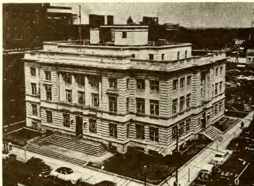
Greensboro Municipal Building
