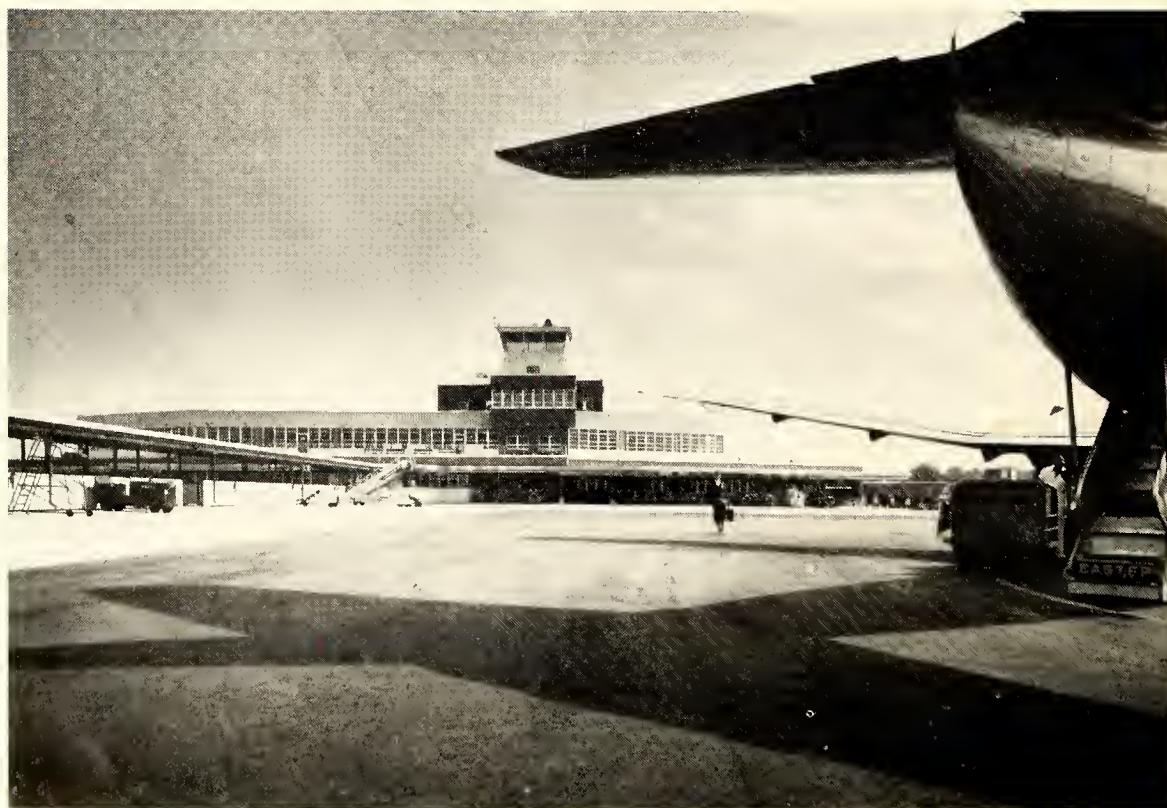
Charlotte Municipal Airport
