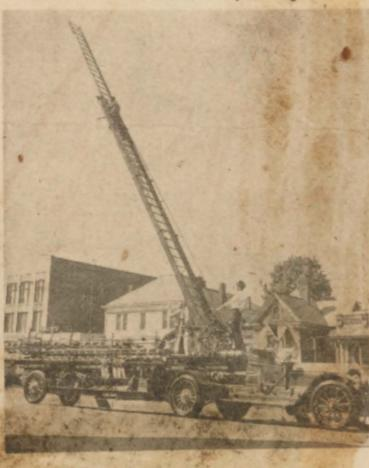
A 60-foot aerial ladder swings into operation during a demonstration by local firemen.
