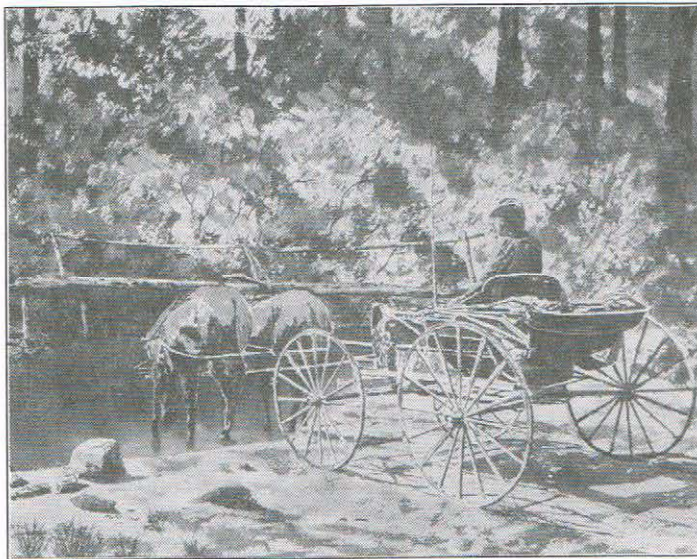
Creek Ford and Footbridge by Samuel D. Bissette
