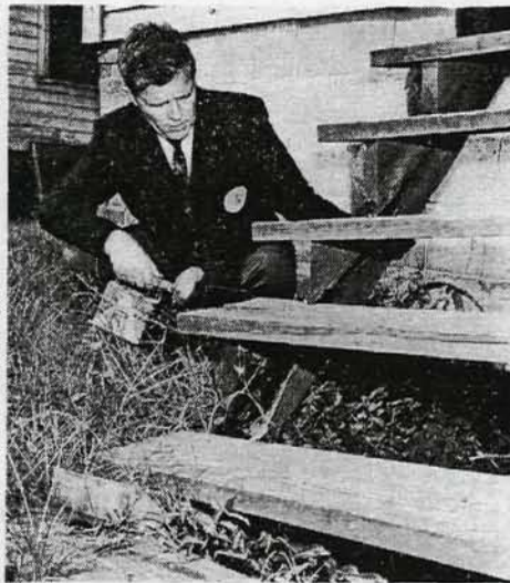
CHECKS FOR CODE VIOLATIONS —John Crabtree, city housing inspector, checks on the condition of a dwelling's porch stairs, left, and its plumbing facilities, right, as part of his regular inspection procedure. The inspections are designed to detect violations of the city's housing code. When violations are found, property owners are asked to make improvements which will bring the dwellings into compliance with the code. Inspections are conducted usually according to a schedule of areas which has been established when the code enforcement program was adopted, although they are often conducted as a result of a complaint about possible violations.
