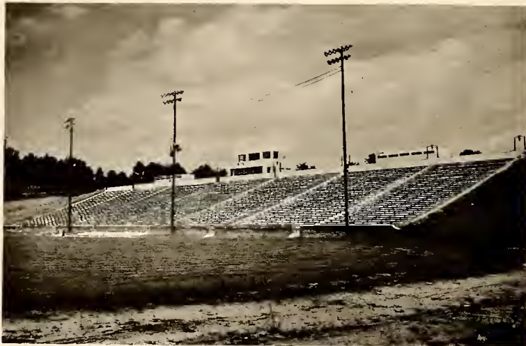
Burlington High School Stadium
