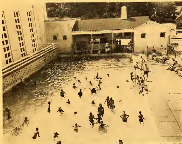
Community Center Swimming Pool
