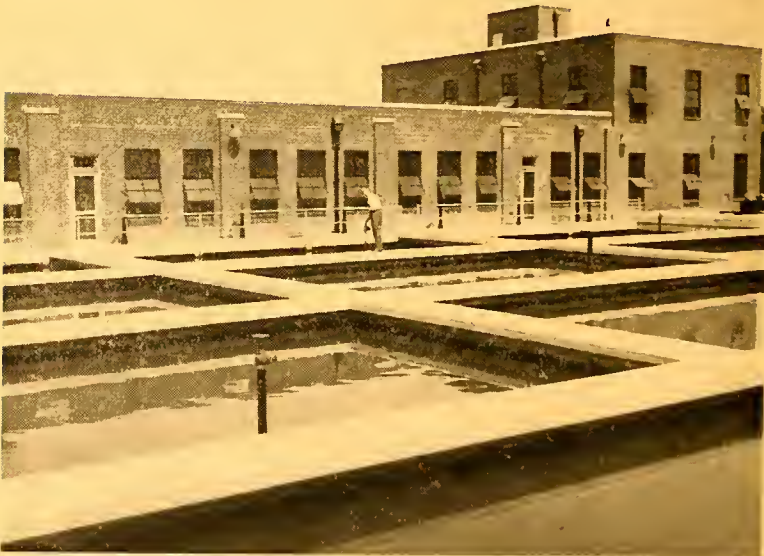
Concord's Modern Water Filtering Plant
