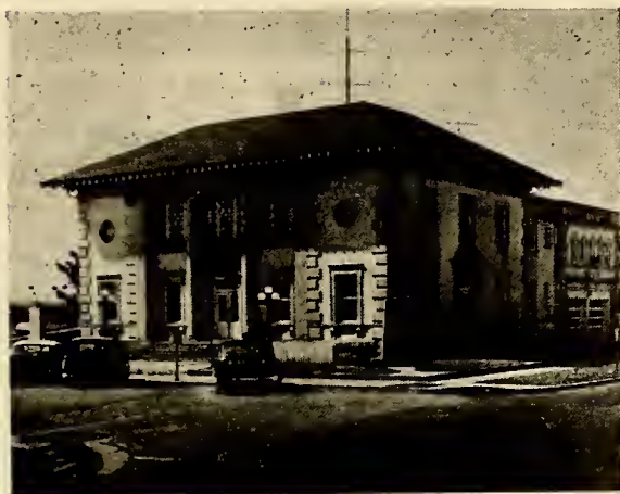
The Morehead City Municipal Building
