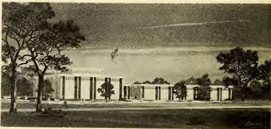
Fayetteville's New Federal Building to house U. S. Court, the Post Office and other Federal Agencies; construction to start early Fall of 1963, completion 1964.
