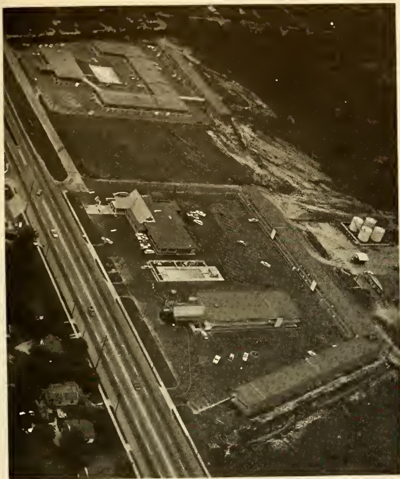
Two of Fayetteville's Thirty Three Motels (1,082 Units)
