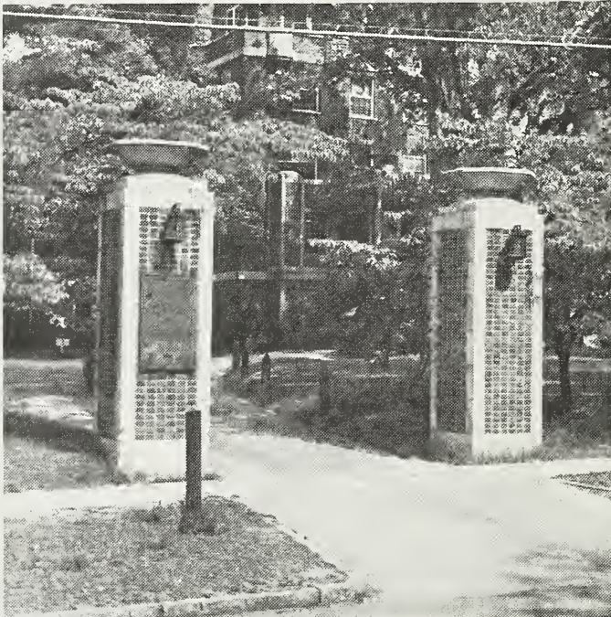
Highsmith-Rainey Memorial Hospital
