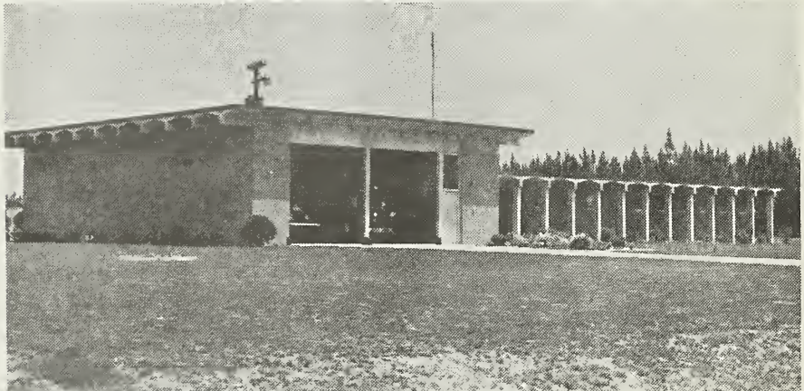
Fayetteville Fire Station No. 5
