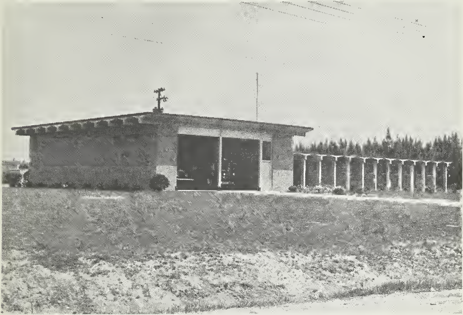
Fayetteville Fire Station No. 5
