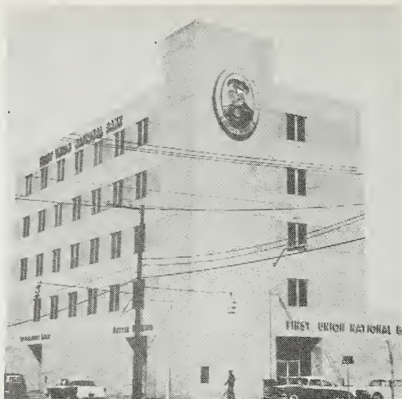
FIRST UNION NATIONAL BANK - 230 Donaldson Street (Downtown), and 4549 Raeford Road. Resources as of December 31, 1963, $439,993,238.33.
