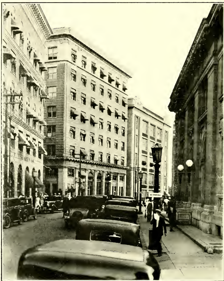
VIEW OF CORCORAN STREET, LOOKING SOUTH
