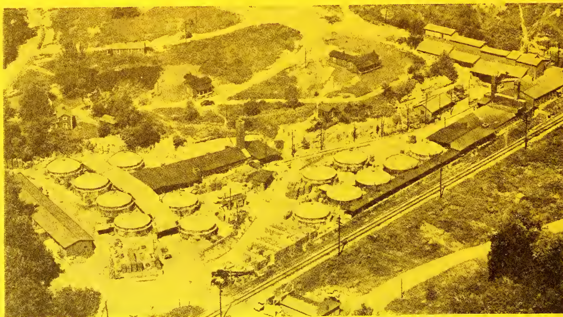
Located in the Pine Hall community a few miles from Winston-Salem, Plant No. 1 supplies Pine Hall Brick for many of North Carolina and Virginia's finest structures. This plant has fourteen round kilns in operation daily.
