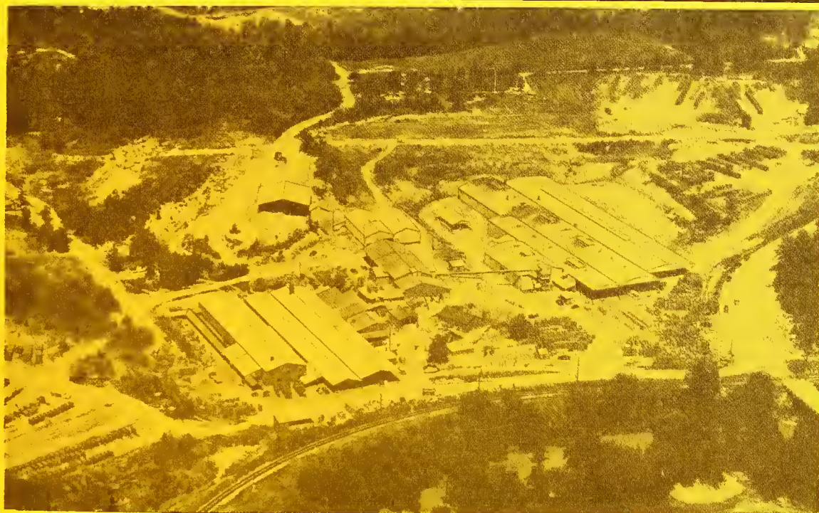
At Plant No. 3, near Modison, N. C., huge tunnel kilns are in operation night and day, producing brick around the clock. Pine Holl's total production is over 650 tons of clay products a day.
