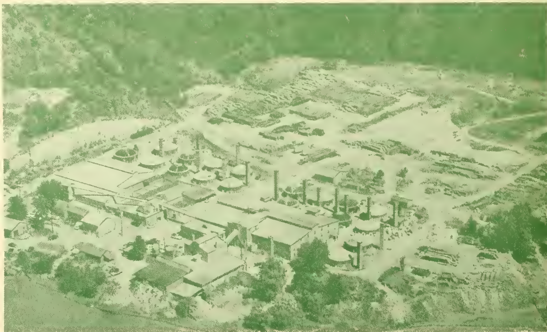
Plant No. 2, a few miles north of Plant No. 1, produces vitrified clay pipe in a variety of sizes.
