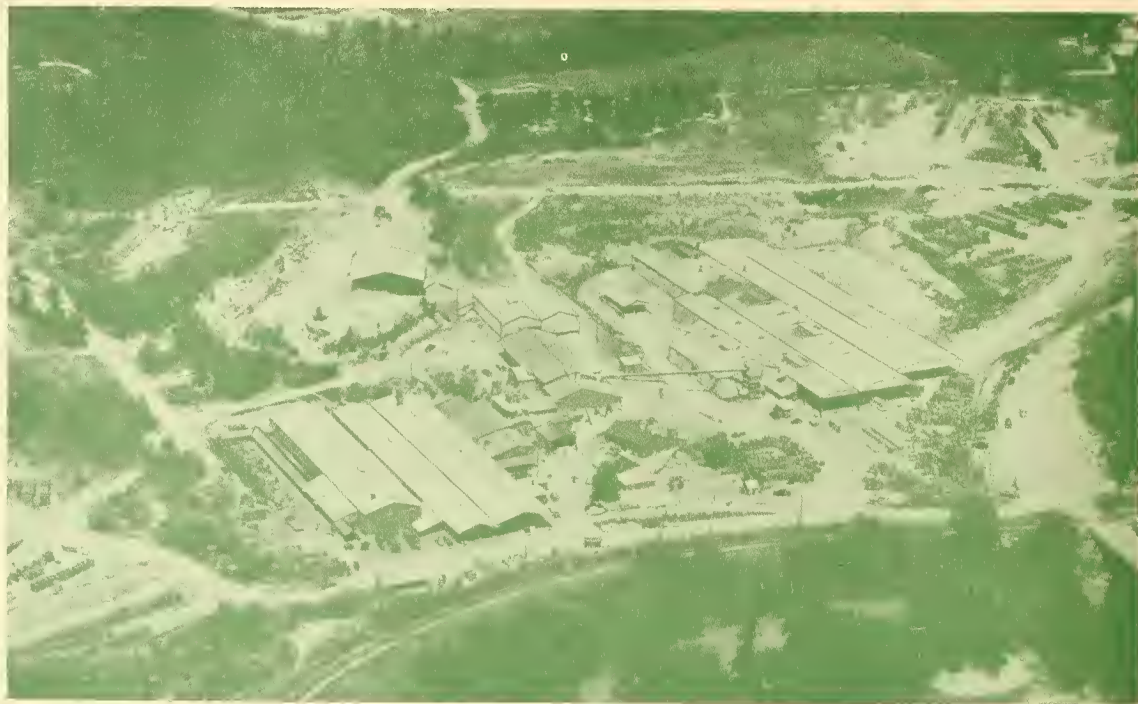
At Plant No. 3, near Madisan, N. C., huge tunnel kilns are in operation night and day, producing brick around the clock. Pine Hall's total production is over 650 tans of clay products a day.
