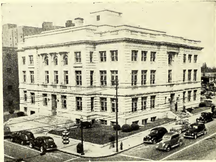
Greensboro Municipal Building
