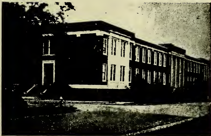
Lee County Hospital, Sanford
