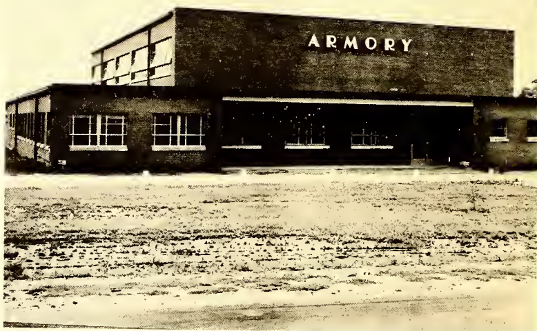
National Guard Armory, Completed in 1955
