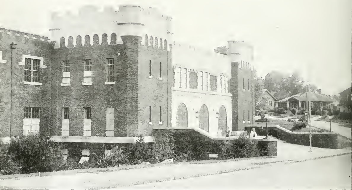
City Armory-Auditorium, Charlotte
