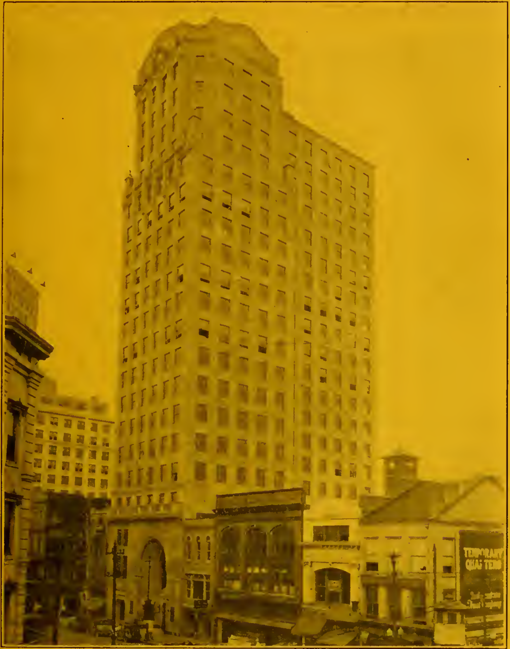
FIRST NATIONAL BANK BUILDING, CHARLOTTE, N. C.
