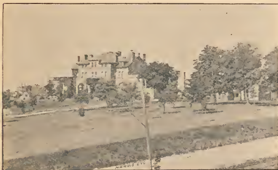
VIEW OF MAIN COLLEGE BUILDING, ETC
