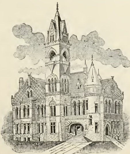
FORSYTH COUNTY'S NEW COURT-HOUSE.
