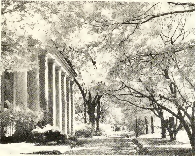
Graham Memorial (The student union building)
