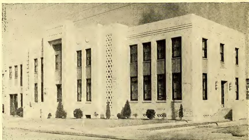
ASHEBORO MUNICIPAL BUILDING
