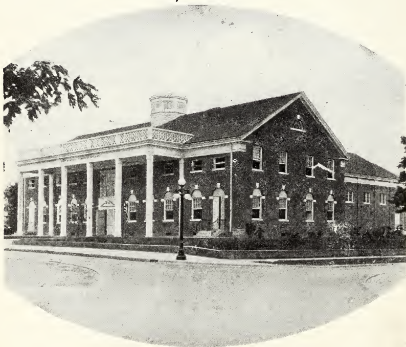
Wayne County Memorial Community Building
