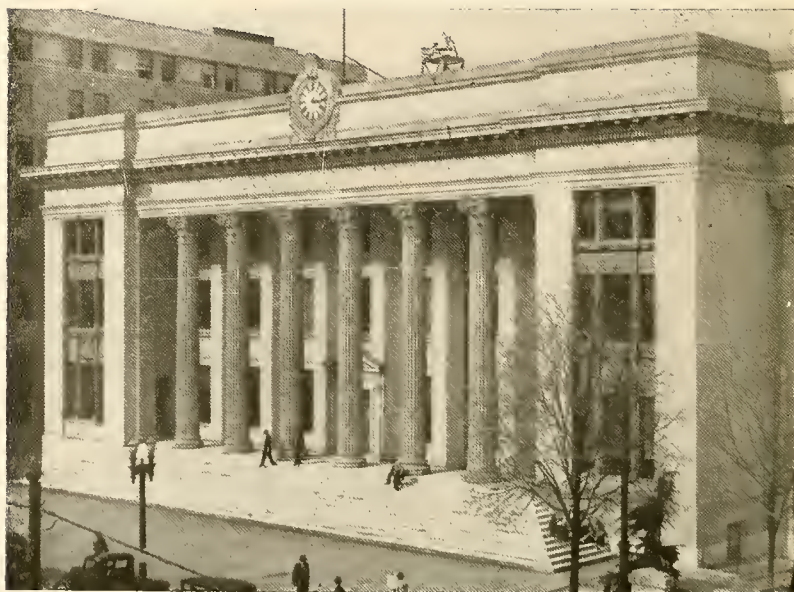
Wilson County Court House
