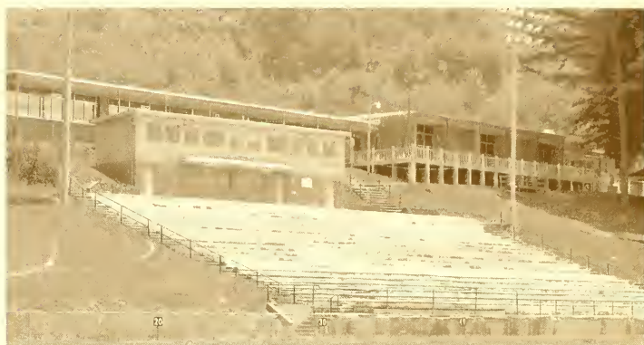
Murphy High School football stadium
